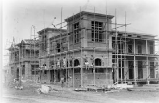
bun01078 Building the Base Hospital ca 1914
