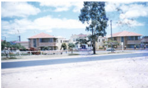
bun01379 Bundaberg Hospital ca1950s
